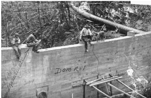
An old dam on the Catawba River
